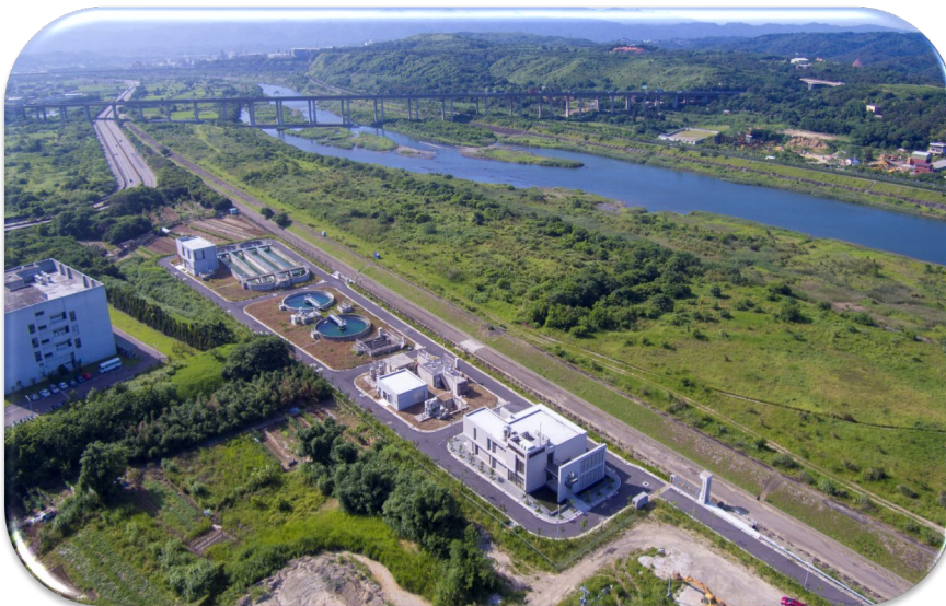
Houlong Township Water Reclamation Centre, Miaoli County
